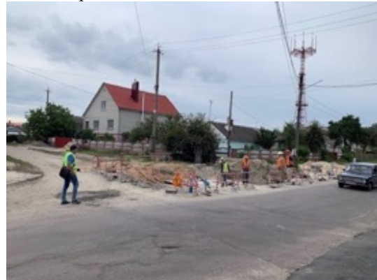
Figure 3 Open pit in an area where the pipe in pipe method is being used, access for cars and pedestrians is uninterrupted
